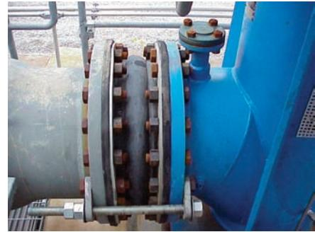
**Figure 1.** Typical elastomeric expansion joint installation.
